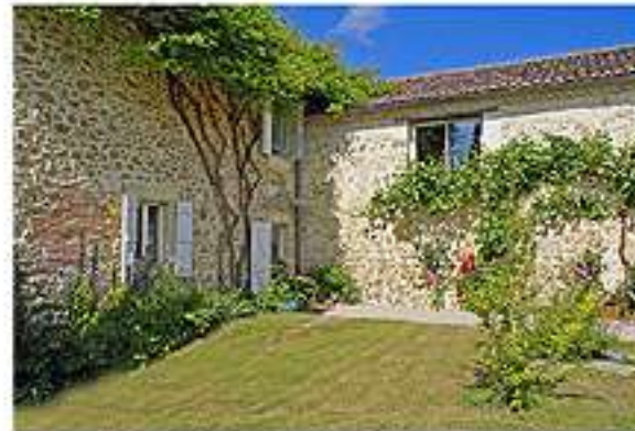
View of the garden before project
